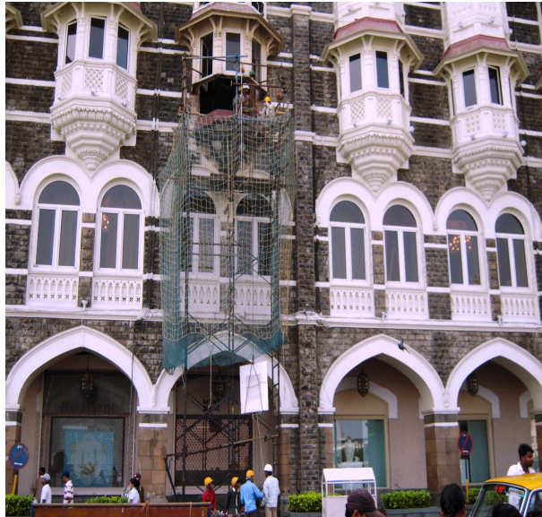
FIGURE (1) BEFORE REPLACING GRC BALCONY (TAJ HERITAGE)
