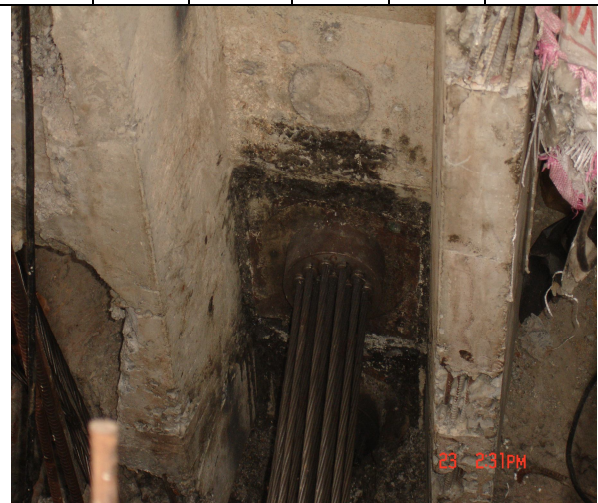
FIGURE (3) CASTING CONCRETE WITH GLASS FIBRE SURROUNDS PRESTRESS STRAND CABLE AT HOLAKAR BRIDGE
