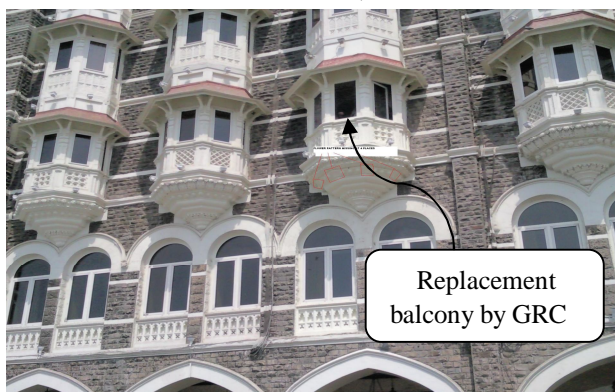
FIGURE (2) AFTER REPLACING GRC BALCONY (TAJ HERITAGE)
